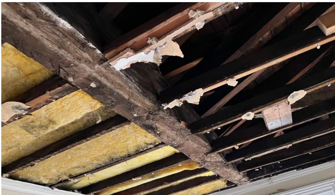
Fig 3: Valley Beam showing Rafters and Ceiling Joists
