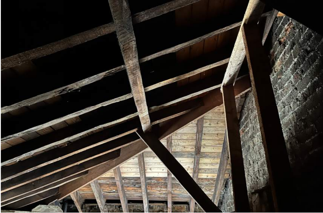
Fig 2: Internal Roof Space showing Rafters, Hip Beam and Purlins
