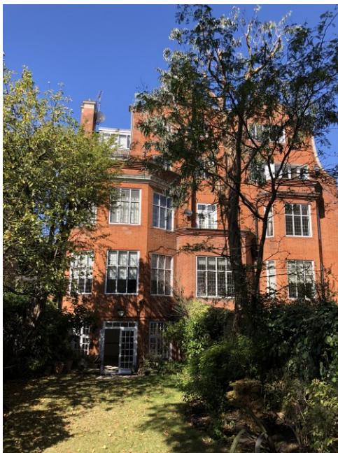
Figure 23 The rear façade of Flat 3 with similarly proportioned French doors in the base of the rear canted bay.
