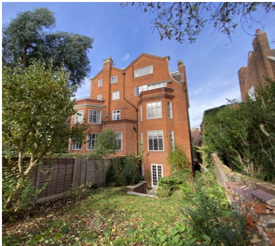
Figure 12 The rear façade of no.39 Eton Avenue and the private garden to Flat 1.
