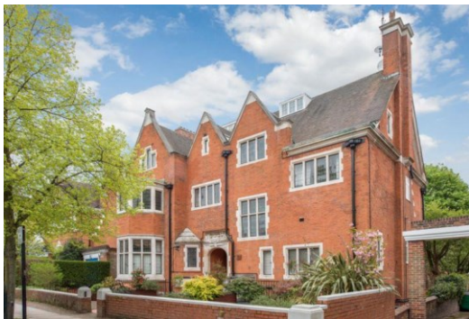
Figure 1 No.39 Eton Avenue.
