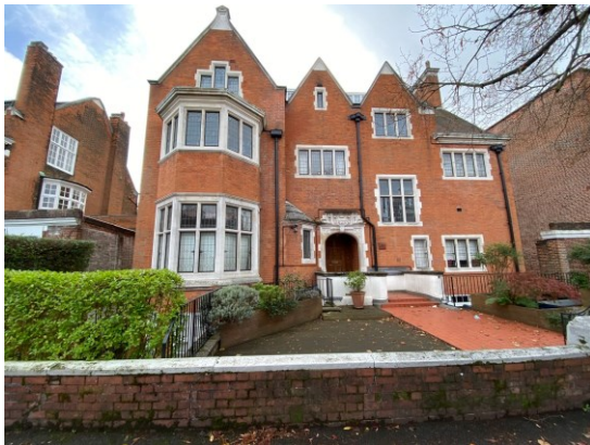
Figure 11 The front façade of no.39 Eton Avenue.
