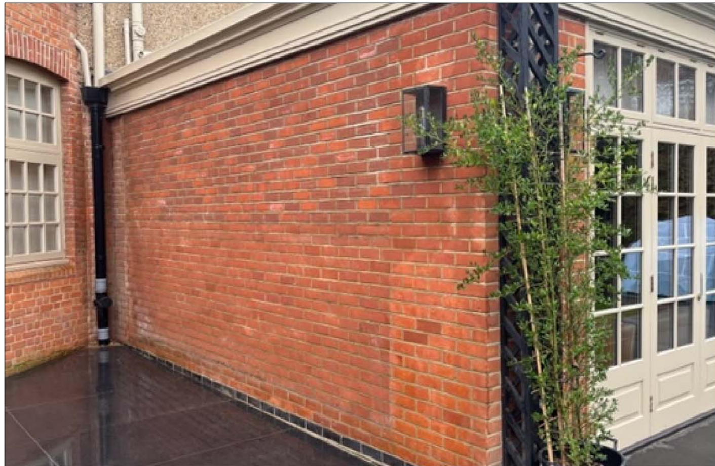
Side of existing extension, 4 Akenside road
