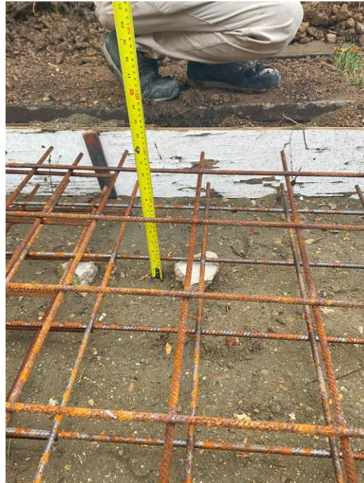
Photograph 4 – RC32/40 concrete and 50mm Bottom cover confirmed. Note cover photo was taken following comments from structural engineer.
