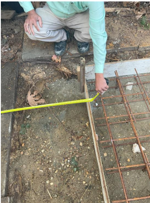
Photograph 2 – Minimum Easement zones to neighbouring retaining walls verified.
