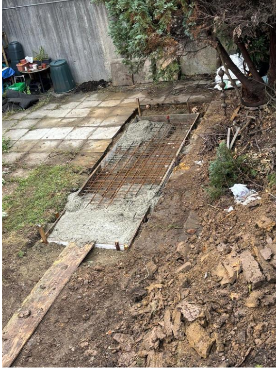
Photograph 5 – Concrete being poured, tamped levelled. Photos courtesy of contractor.
