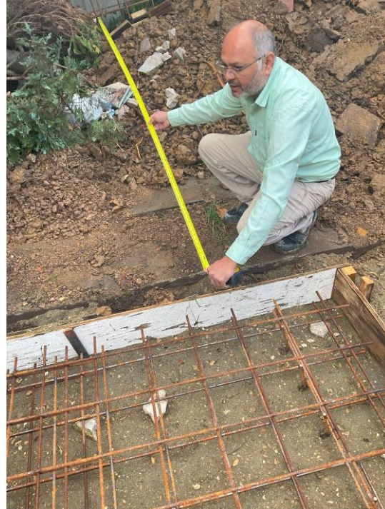
Photograph 2 – Minimum Easement zones to neighbouring retaining walls verified.
