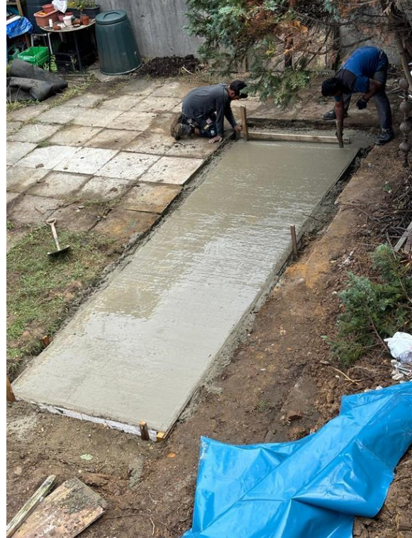
Photograph 5 – Concrete being poured, tamped levelled. Photos courtesy of contractor.
