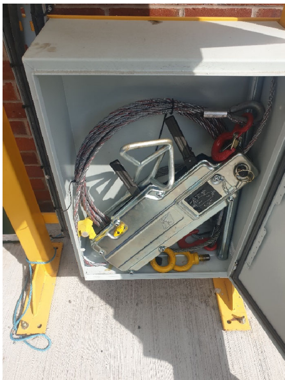
Figure 30 Emergency manual rotation kit
