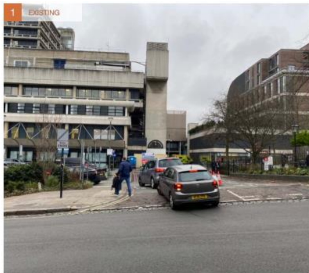
Pond Street Entrance - existing
