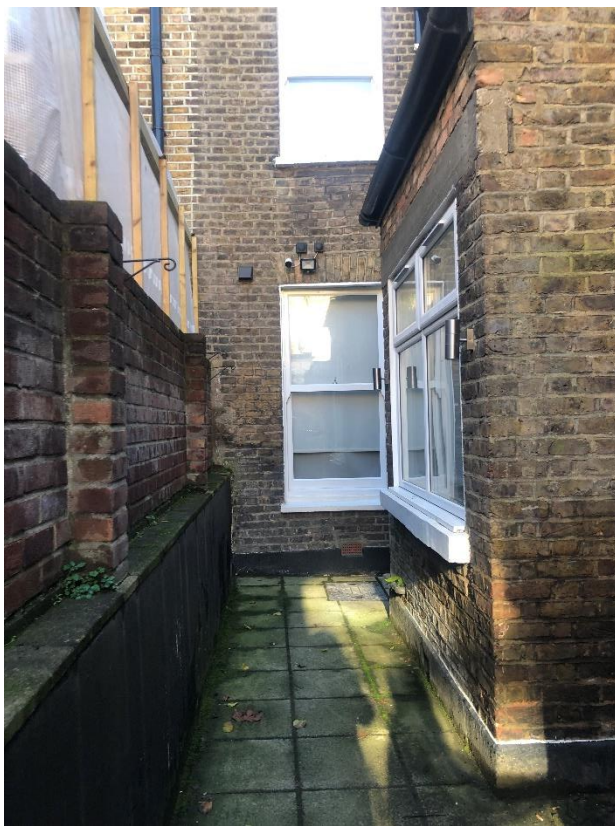
6. View of the side garden and boundary with no. 91.
