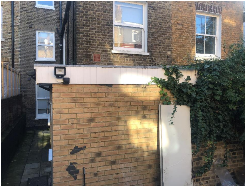
3. Rear view of the property and single storey rear extension.
