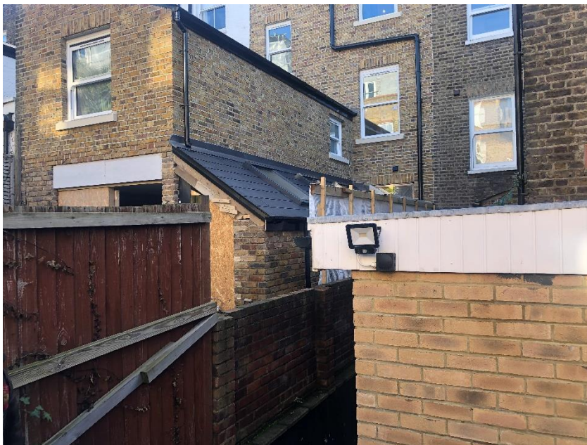
4. View from the rear garden, of the rear extension towards no. 91.
