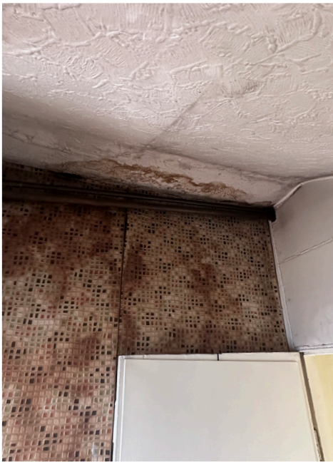
Leaking roof in store room
