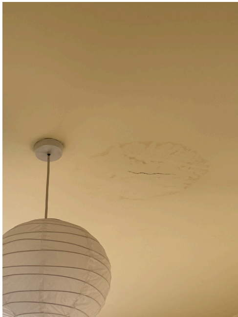
Leaking roof in bedroom 2
