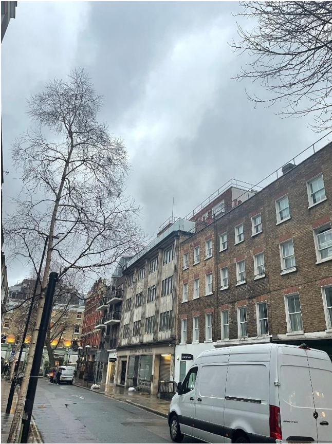
Figure 1: The application site (centre) as viewed from the intersection of Whitfield Street and Windmill Street. The proposed caravan would be set behind the frosted glass balustrade.
