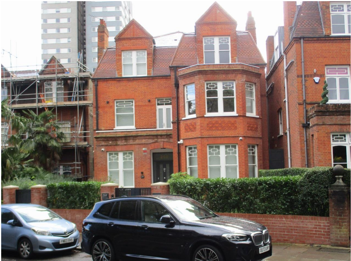
Picture 1: Current front garden with no sign of any trees (1 st Oct. 2024). T1 on the agents application diagram would be on the far right side near the front boundary, but it has long-since been removed.
