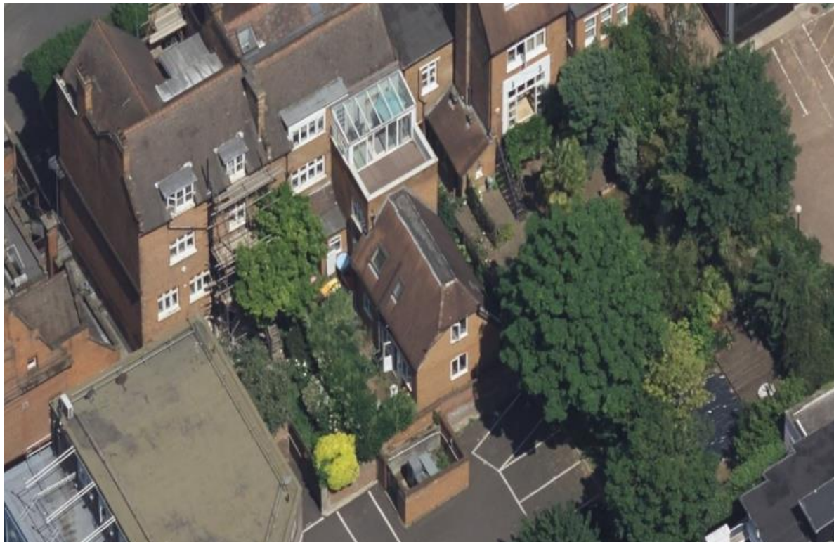
Figure 6 – Aerial view of The Garden Cottage, 2 Netherhall Gardens
