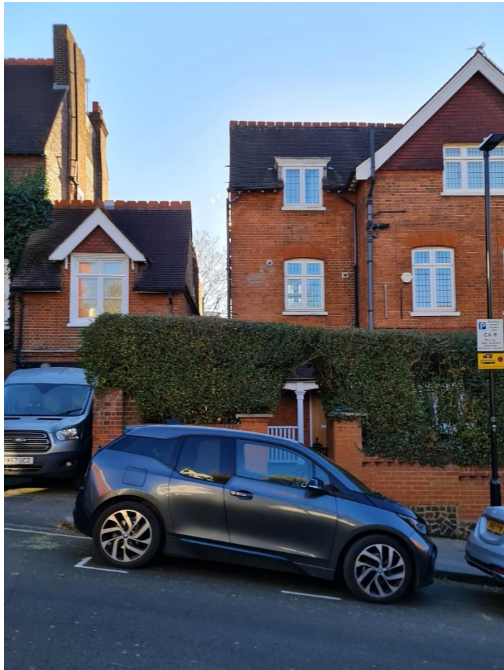
Figure 4 – View from Netherhall Gardens
