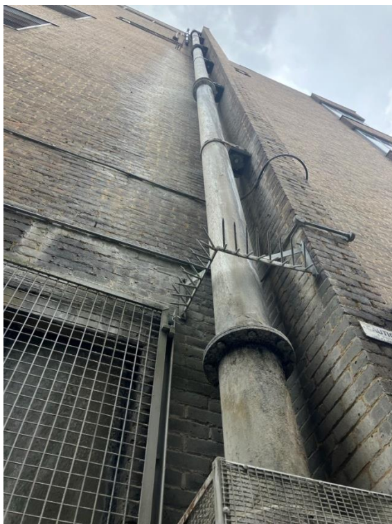
Figure 1: Existing extract flue, image taken from ground floor level.
