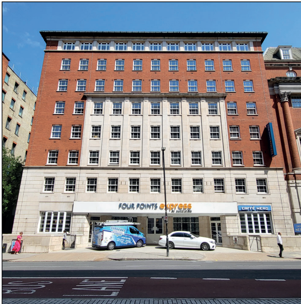
Fig. 7. County Hotel, Upper Woburn Place (July 2024)
