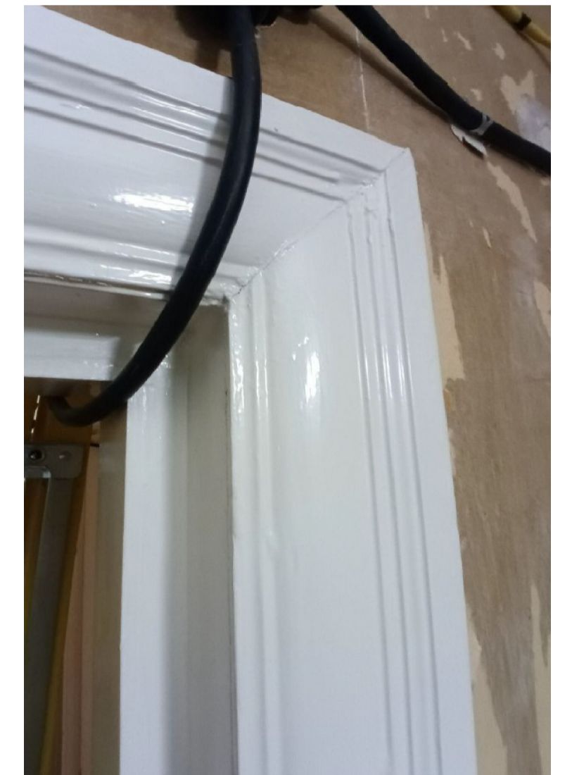
ARCHITRAVE PROFILE IND-110-GF-02 K/L/D Room (All ground floor doors excluding flat entrance) scale 1:1
