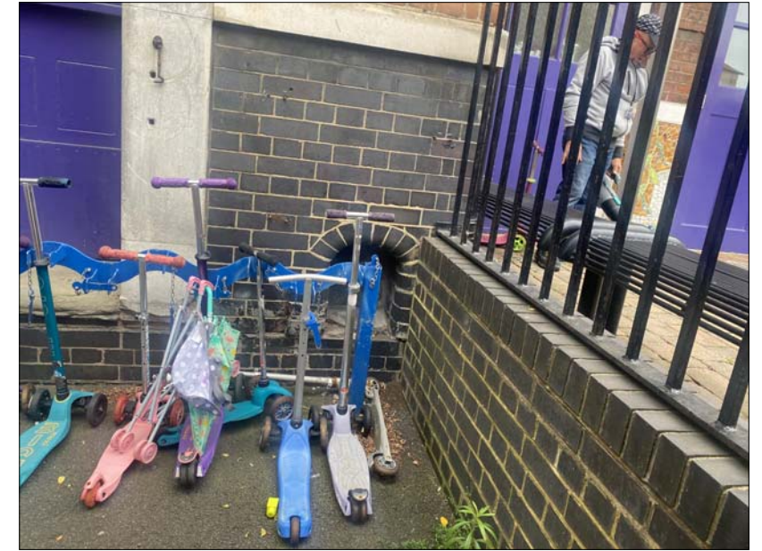
Recess for boot scraper to be retained.
