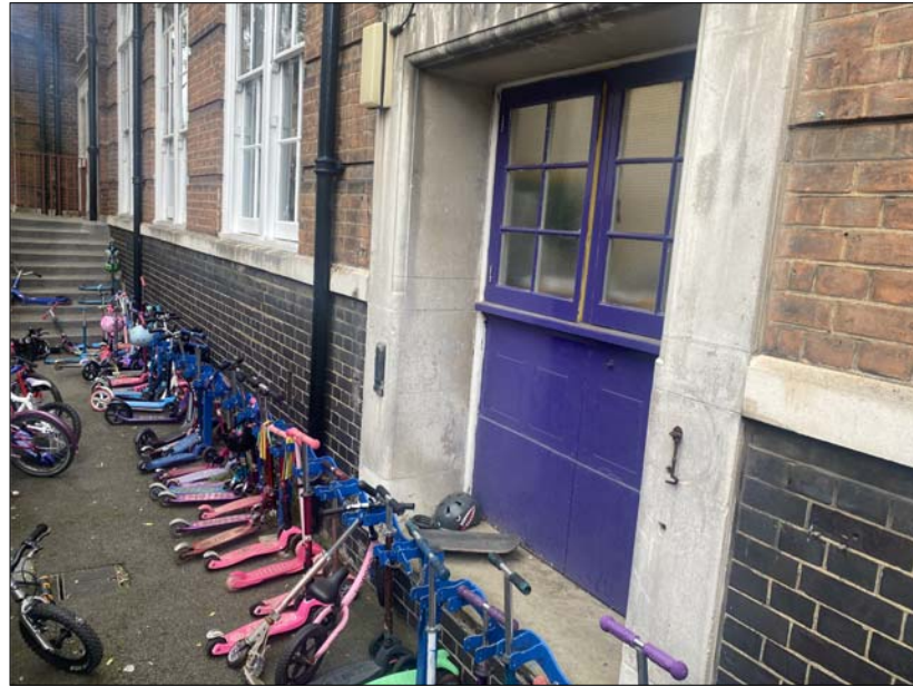
Timber glazed screen to be replaced.
