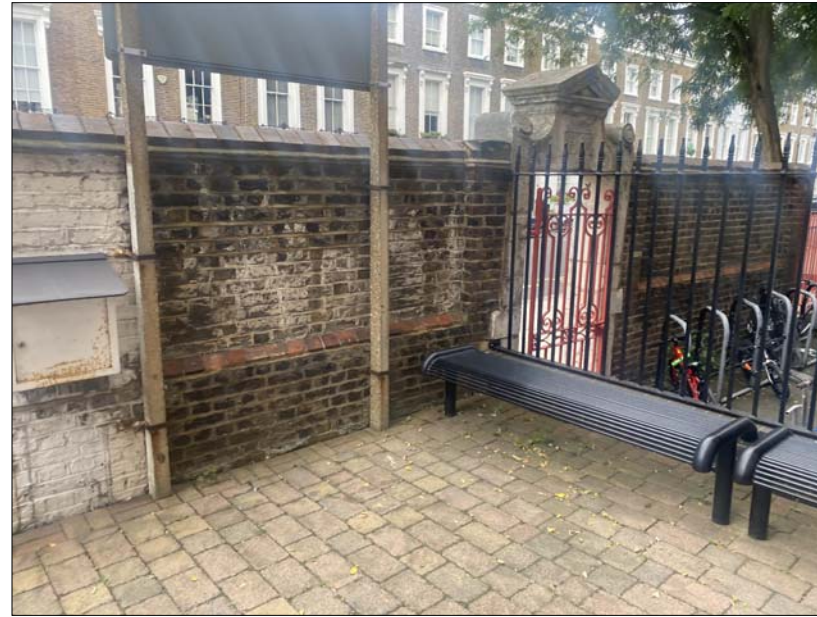
Metal fence to be relocated.
