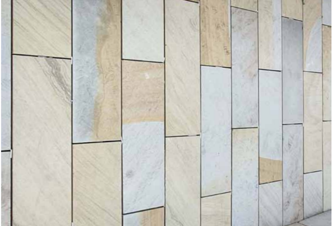
SP6B - Stone colour sample (slope ramp view) Setting out pattern as per sizes above & landscape paving drawings
