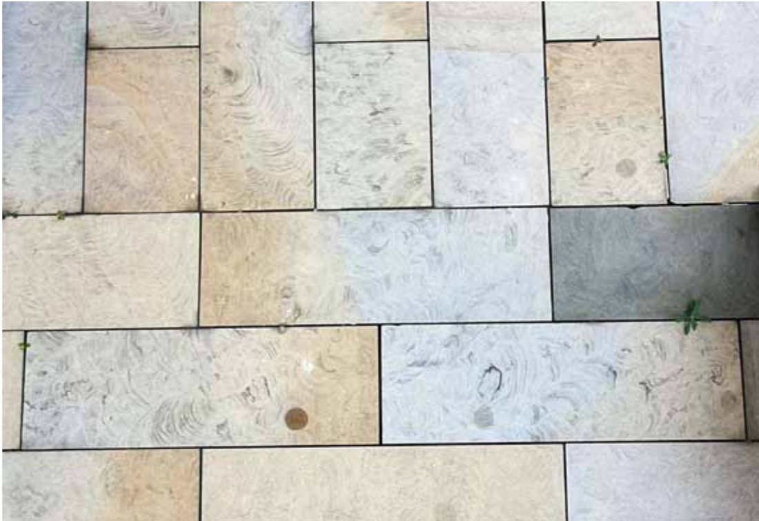
SP8 - Stone colour sample - alternative setting out pattern Setting out pattern as per sizes above & landscape paving drawings
