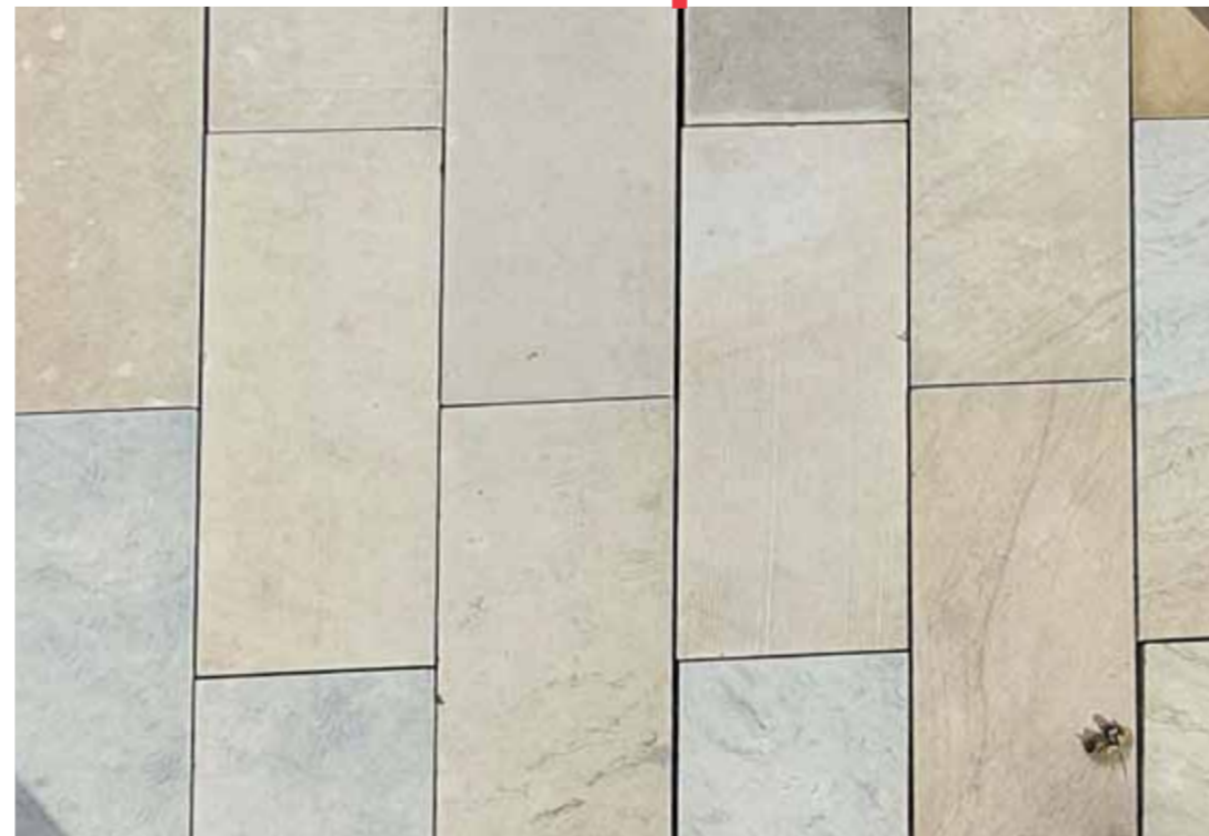
SP6C & SP6D - Stone colour sample Setting out pattern as per sizes above & landscape paving drawings
