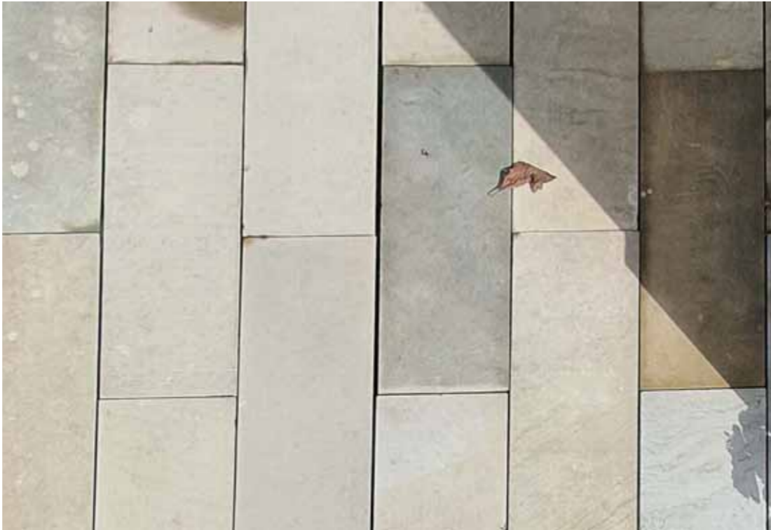
SP8 - Stone colour sample daylight & shadow view of stone. Setting out pattern as per sizes above & landscape paving drawings
