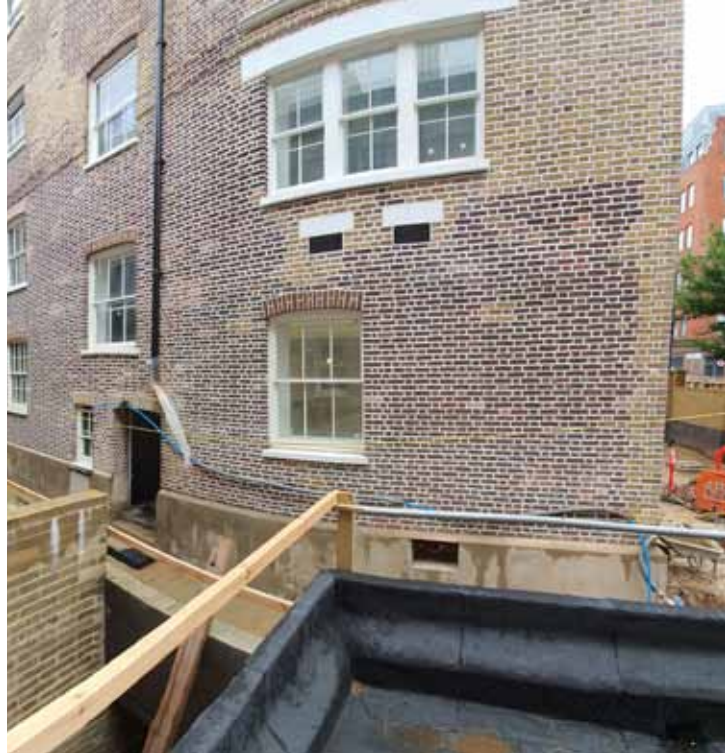
The workhouse consists of yellow stock and red bricks.
