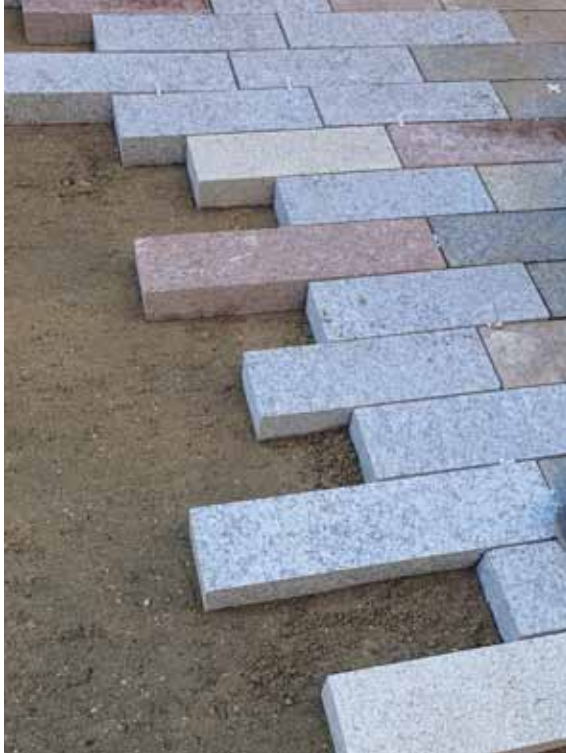
Sample laid out on site to show mix of granite Setts.
