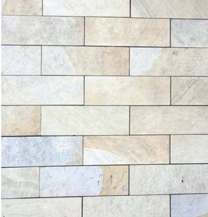
Material SP1 Workhouse entrance ramp - Yorkstone Paving
