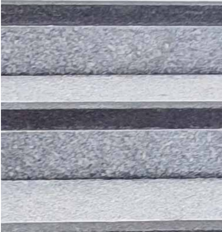
Material ST area - Marshalls Granite steps
