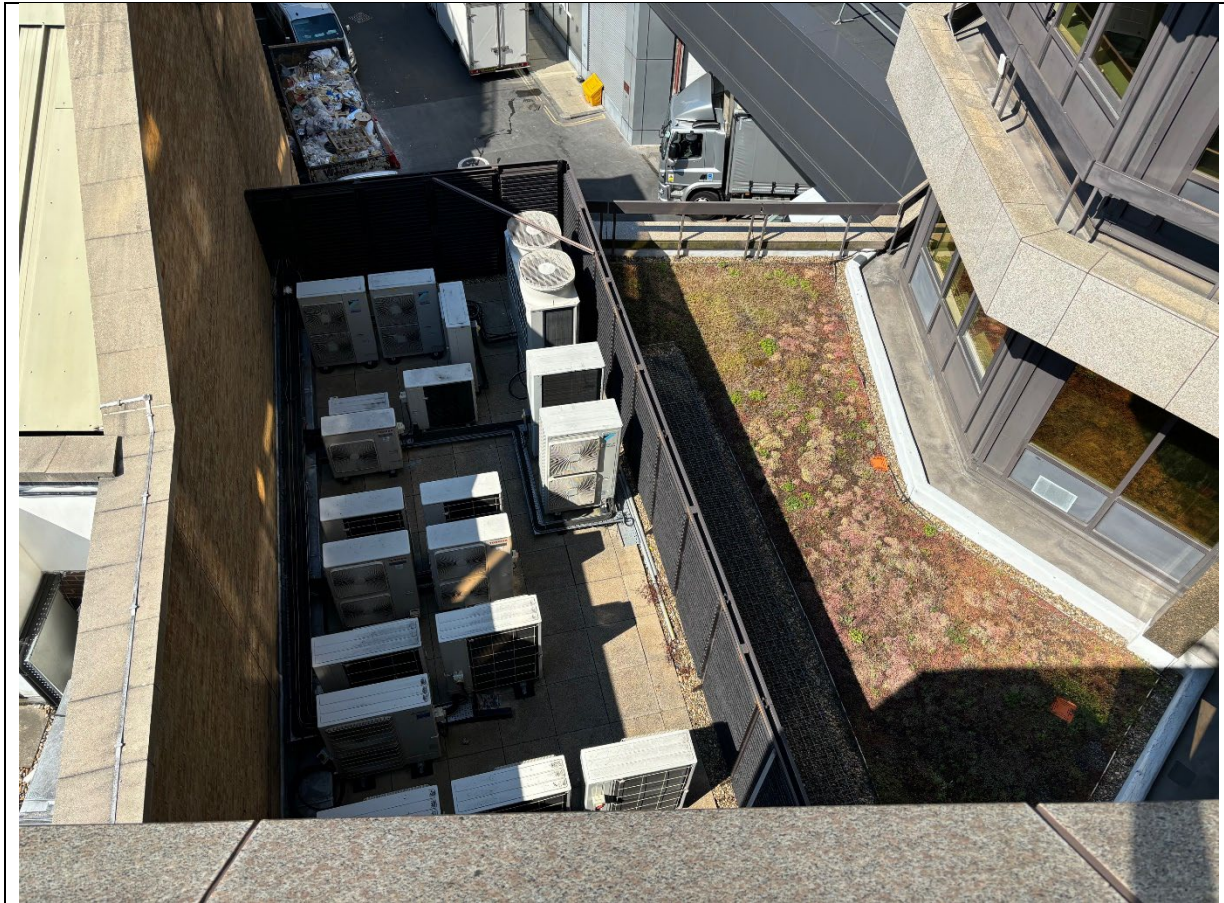
Figure 1: Roof plant area 1
