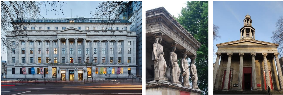
Photos of the Welcome Institute and St Pancras Church within Bloomsbury Conservation Area
