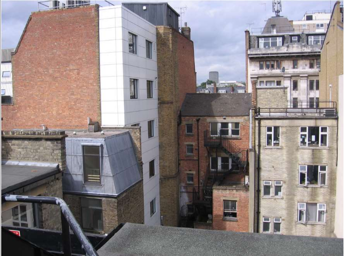
Rear view of 44 (white façade on L), 45 (red brick C), and 46 (R) Hatton Garden (looking west)
