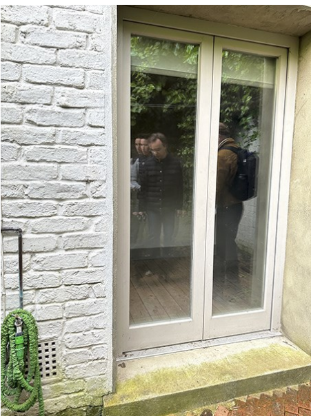
Fig.8 lower ground existing patio doors
