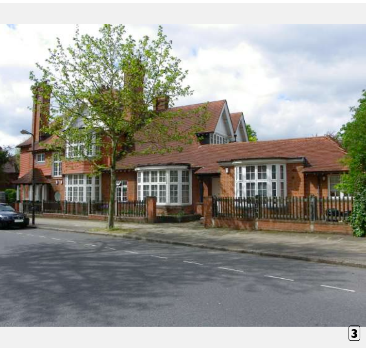
EAST-MAIN FACADE - WADHAM GARDENS
