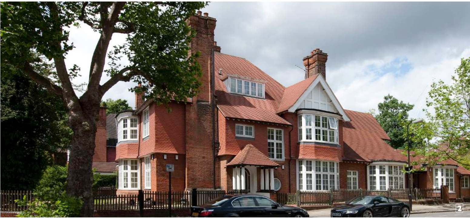
EAST-MAIN FACADE - WADHAM GARDENS
