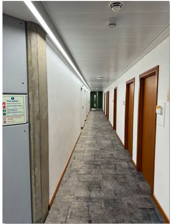
Typical corridor view across 2 nd , 3 rd & 4 th floor corridors - post refurbishment (2022/5402/L) New FD30 flush panel doors, stained finished to match refurbished retained door frames, architrave & skirting
