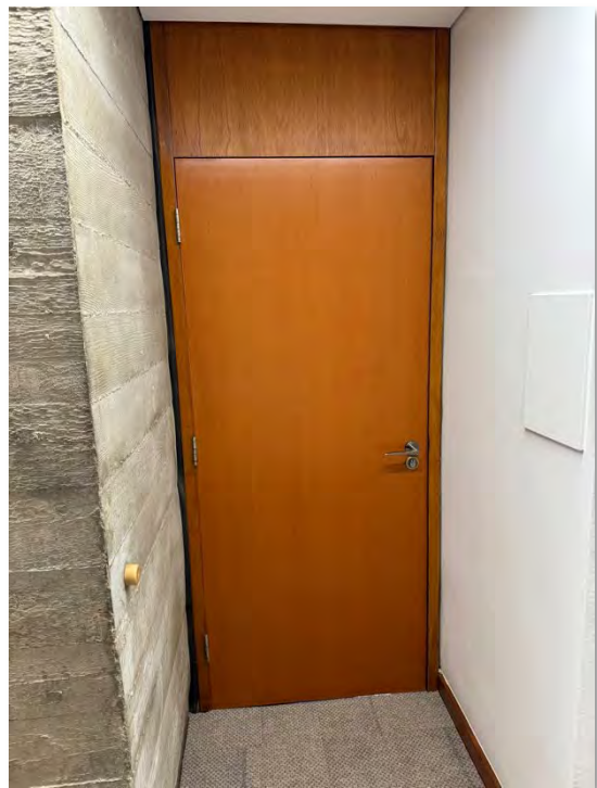
New FD30 flush panel door with fixed panel over, stained finished to match refurbished retained door frames, architrave & skirting
