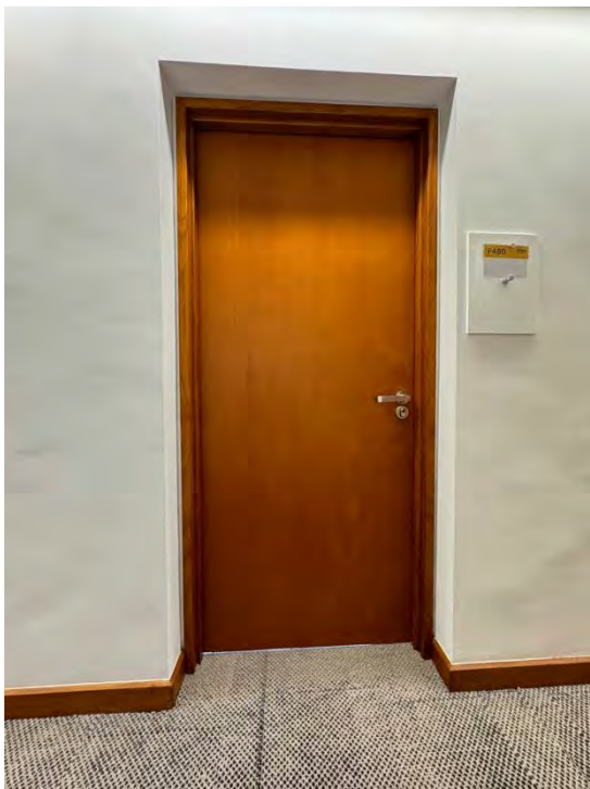
New FD30 flush panel door, stained finished to match refurbished retained door frames, architrave & skirting
