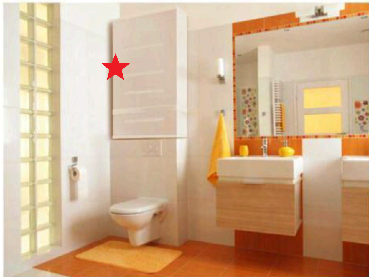
Vertical hot water tank above suspended WC
