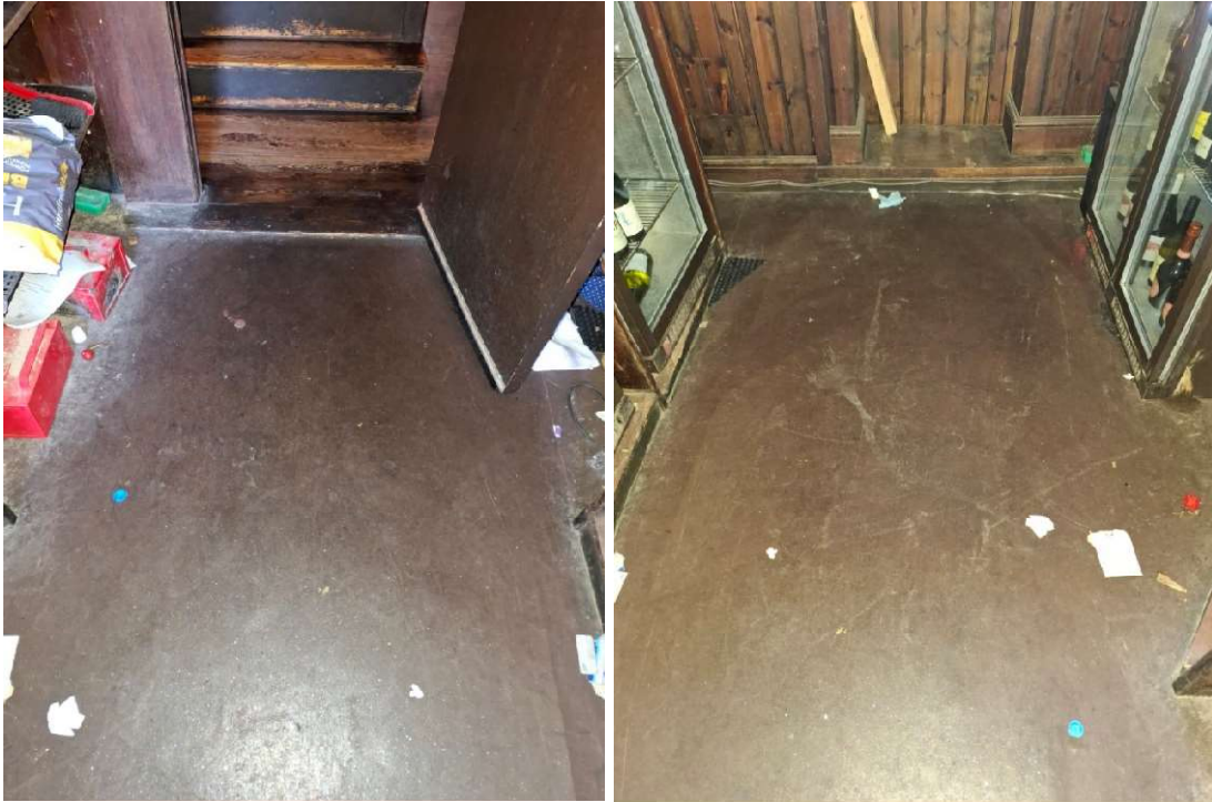
12. Existing altro (vinyl) safety flooring to be removed and new timber floor boards to be laid. New floor boards to be butted up to existing timber threshold and skirtings.
