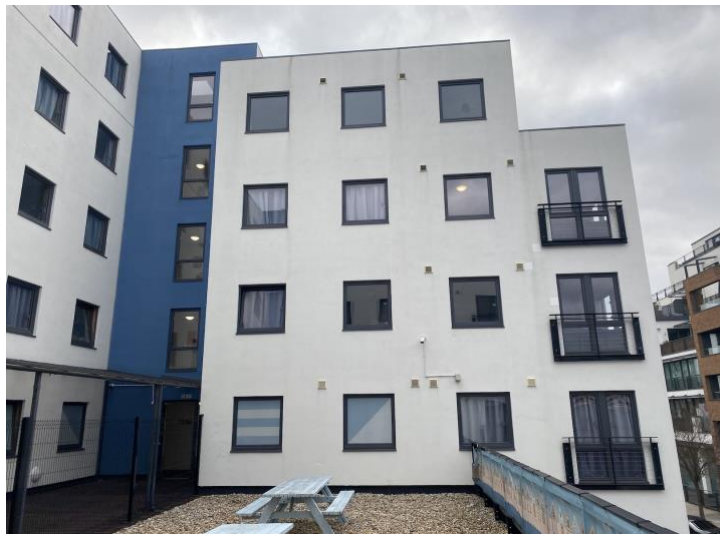
Image from First floor Terrace area – 3.
