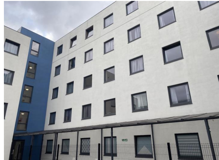
Image from First floor Terrace area – 2.
