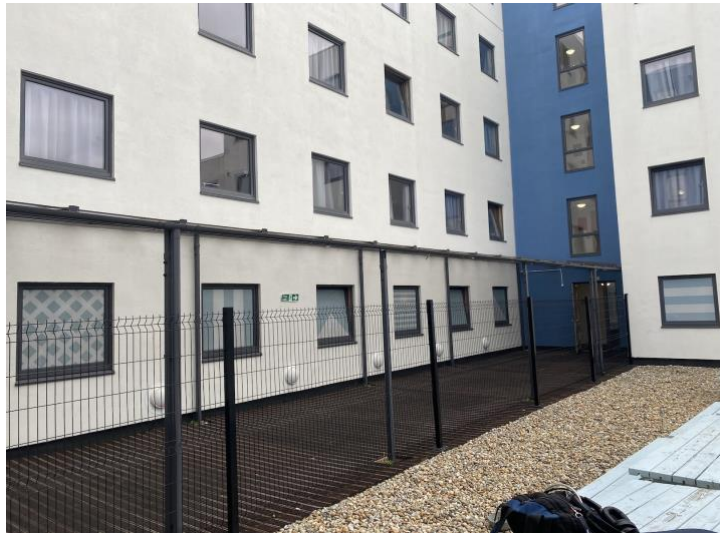
Image from First floor Terrace area – 1.
