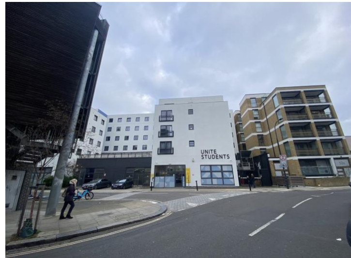
Front Elevation / Main Entrance to Mary Branker House.
