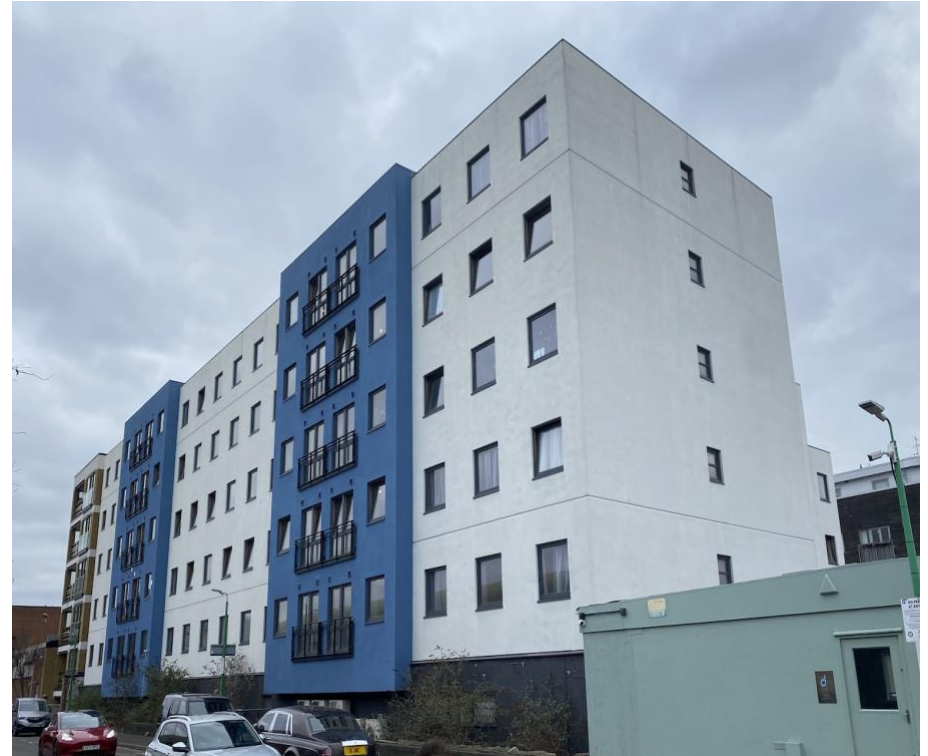
Rear Elevation of Mary Branker House from Regis Road - 2.
