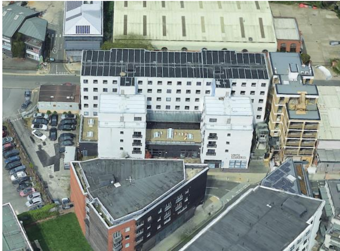
Aerial view of Mary Branker House.
