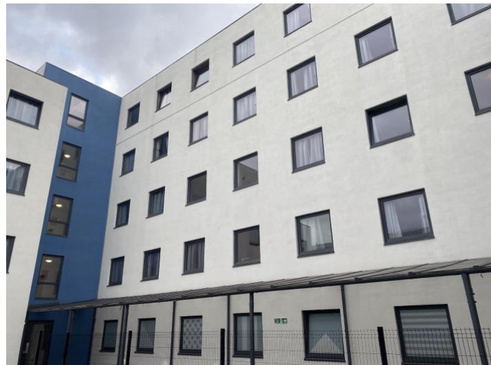
Image from First floor Terrace area – 2.
