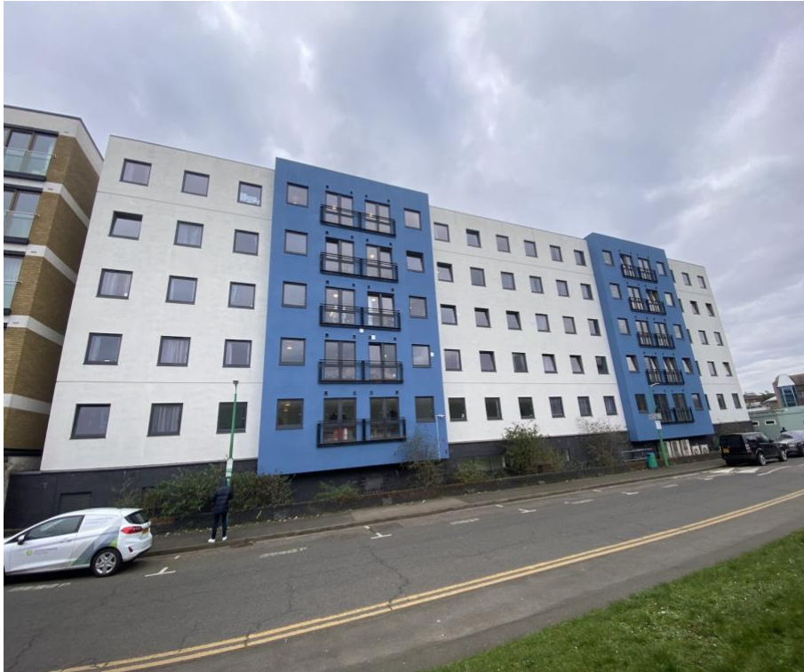
Rear Elevation of Mary Branker House from Regis Road - 1.
