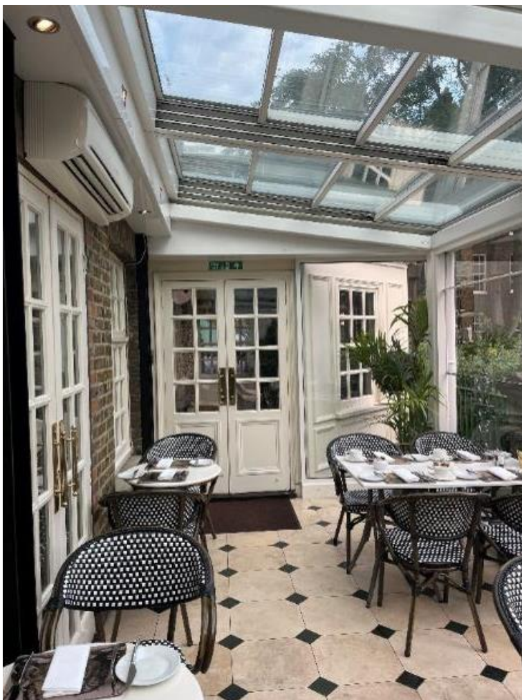
Plate 12: Existing single-pitched glazed element when viewed from within.
