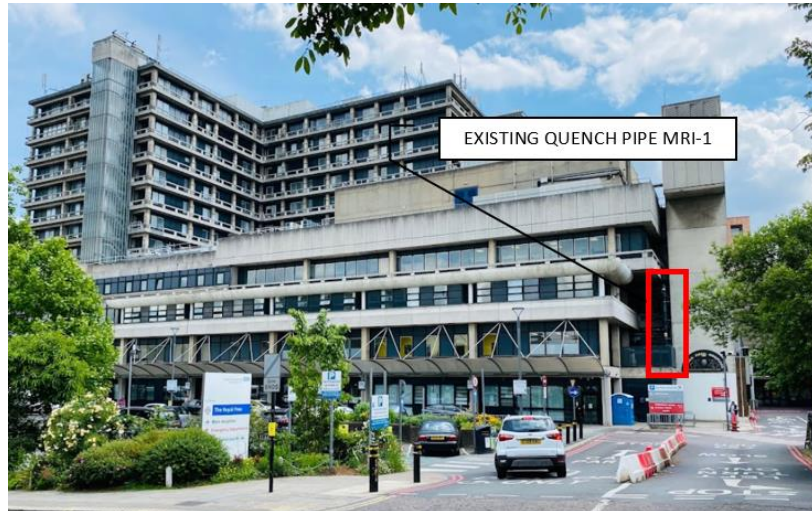
Image 3. MRI-1 Quench pipe. View from Pond Street facade
