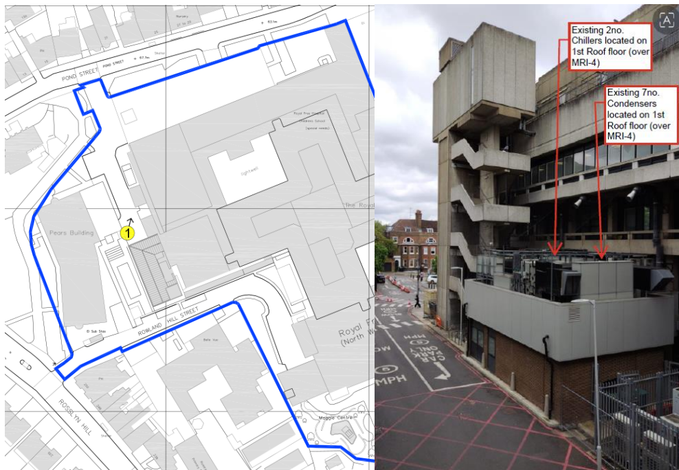
Image 1. Temporary relocation of 2no. Chillers & 7no. condensers. Current location of these units
