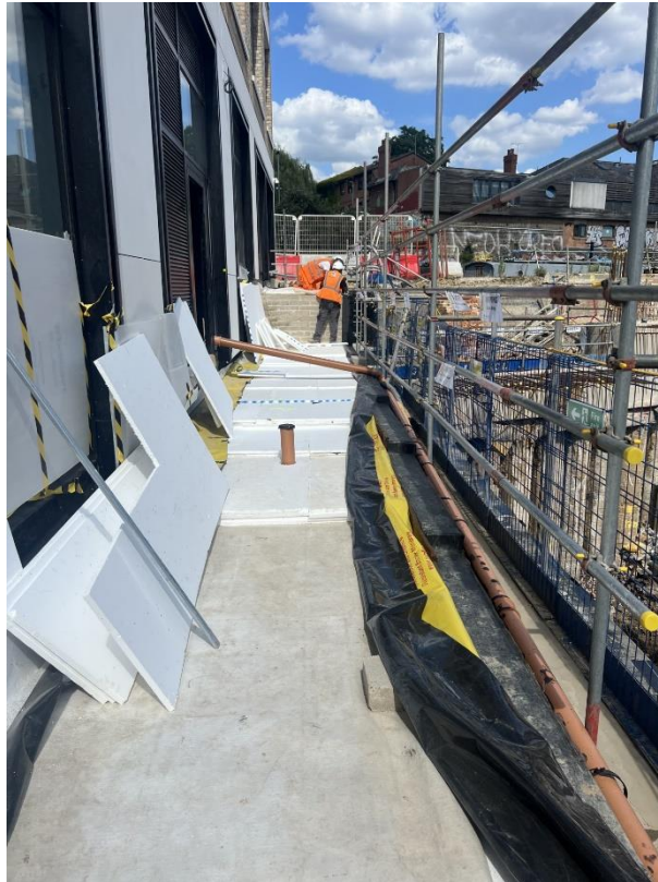
VOC MEMBRANE TO ENCASE FILCORE SYSTEM ON TOP AND ALL VERTICAL FACES
