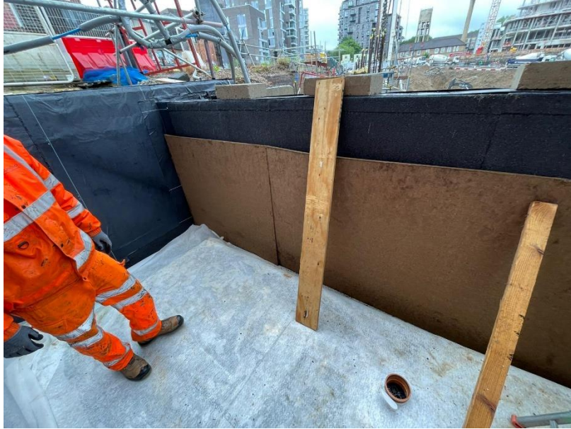
18mm Flexcell expansion joint between retaining wall and tank
