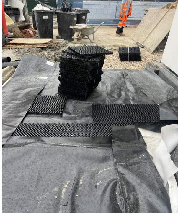
60mm roofbloxx wrapped in GEOMEMBRANE LAYER
