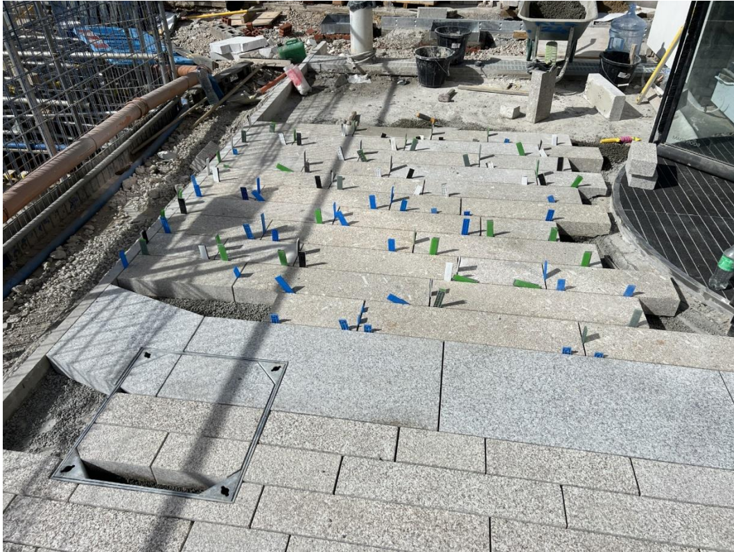
Paving (Permanent – 80mm block and 30mm mortar)
