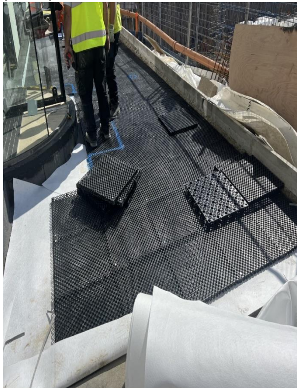
30mm Roofbloxx wrapped in protection fleece at low level
