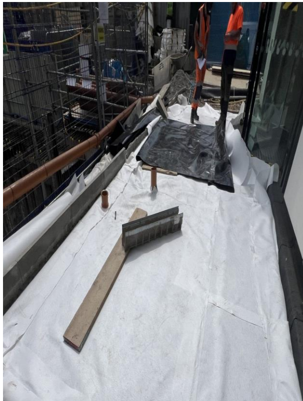
ACOTex PLUS GEOTEXTILE PROTECTION FLEECE INSTALLED OUTSIDE ACOWRAP SYSTEM
