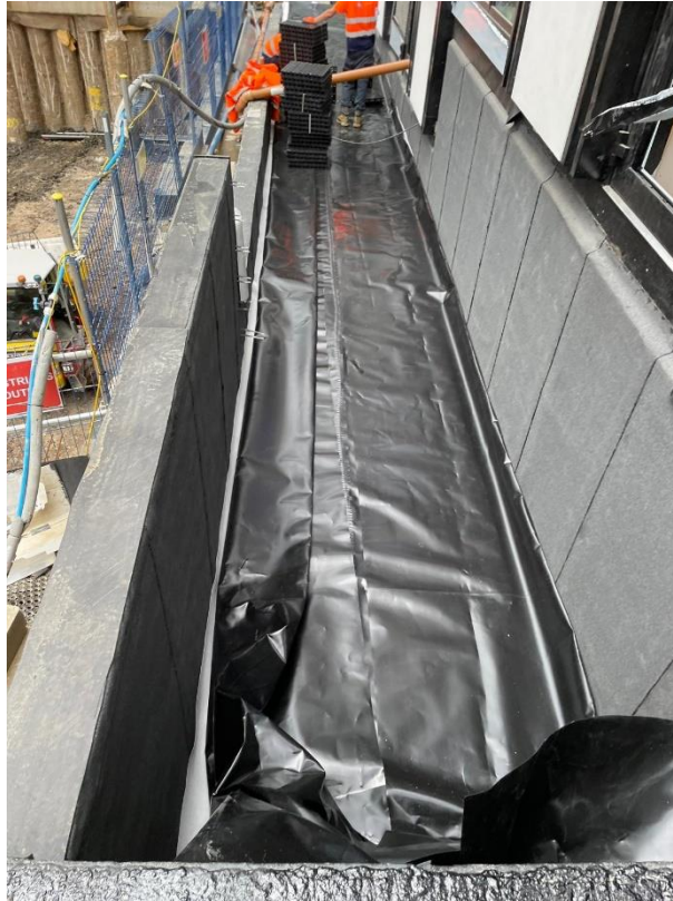
195mm HIGH ACO ATTENUATION TANK wrapped in GEOMEMBRANE LAYER (Initial 1.5m constructed 165mm high)
