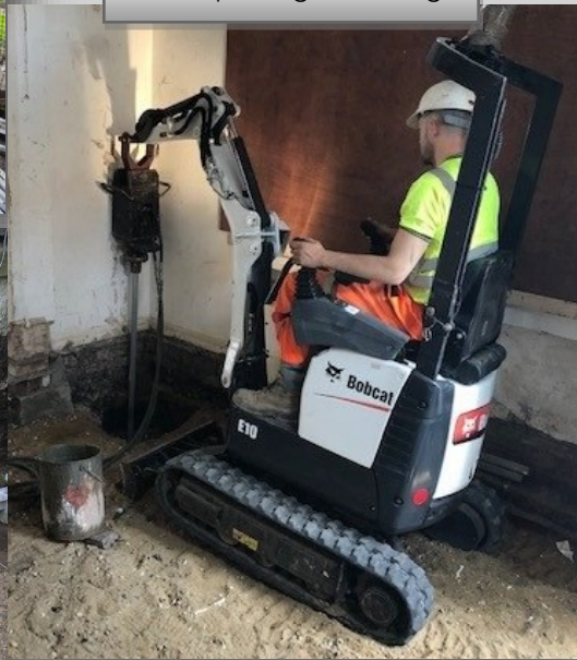
Underpinning a building
