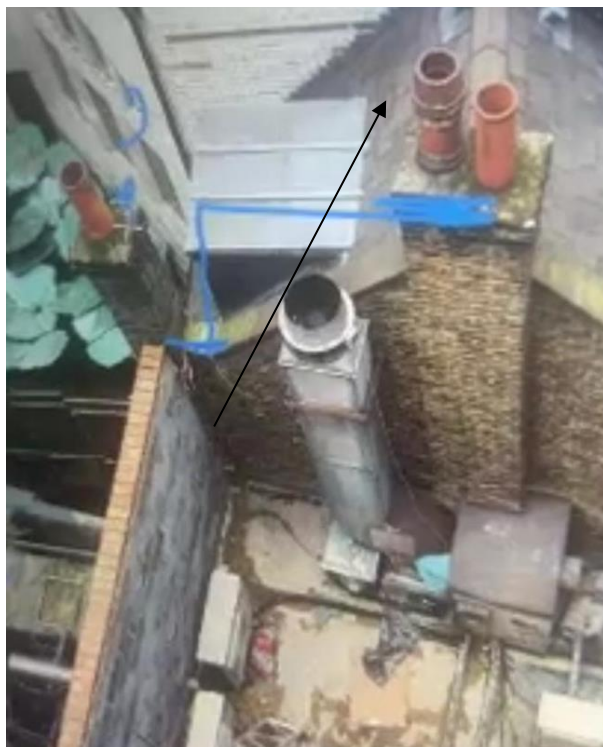
Figure 3 Photograph of Original Flue
