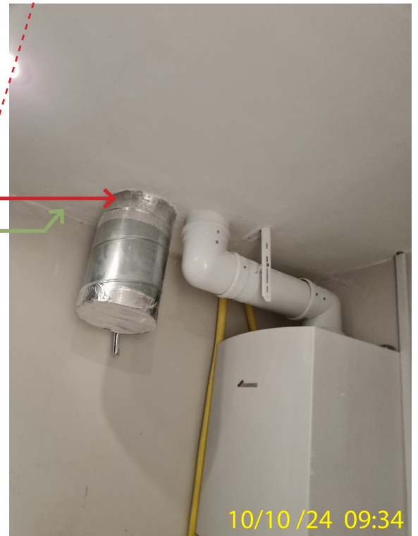
Photo of duct work completed on site. Note: supply duct terminates in ceiling void behind finishes and therefore not visible. Taken on 10th October 2024
