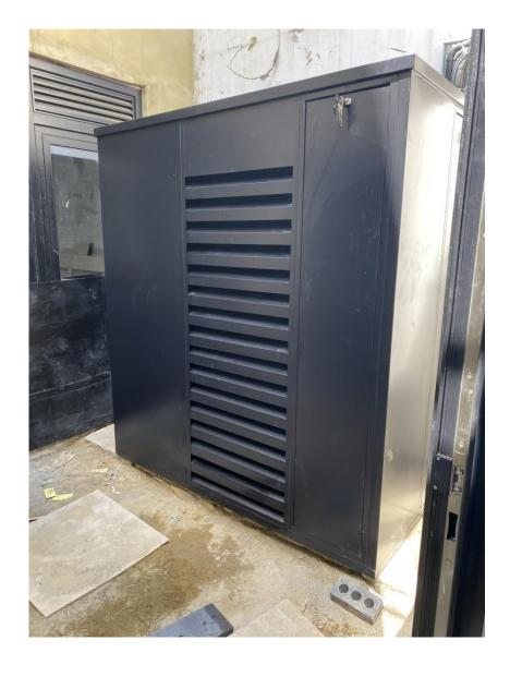
Figure 3 – Typical Acoustic Enclosure 76 Southampton Row, London WC1B Project 13897
