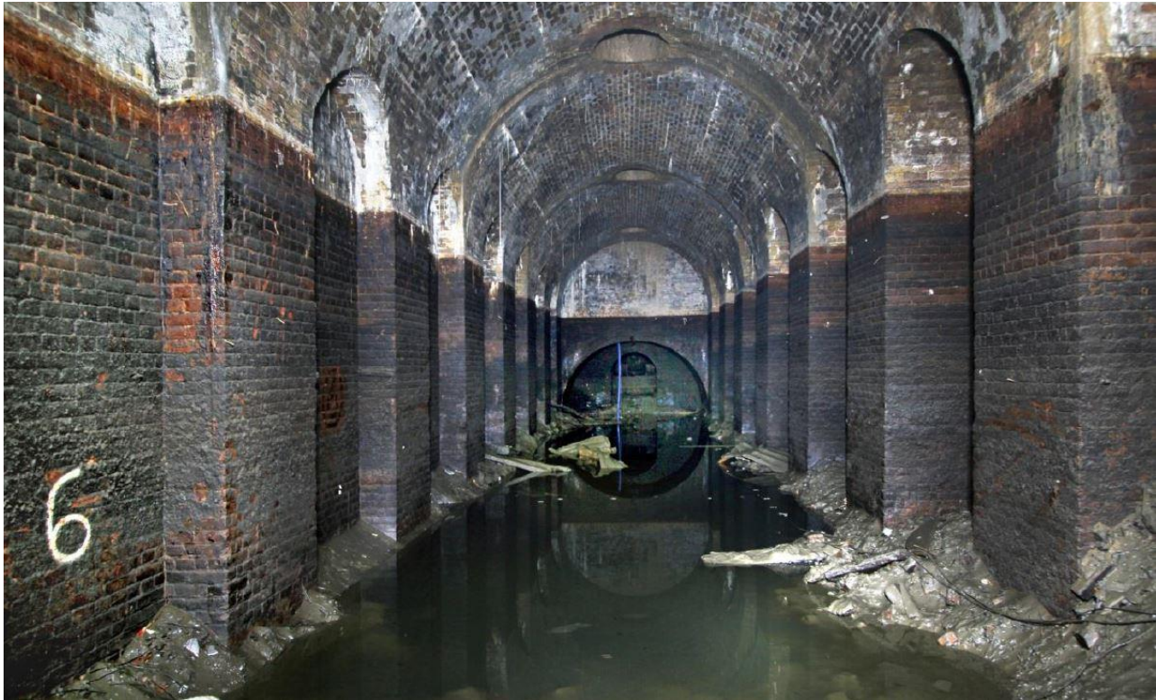
Figure 9 – Flooding in the tunnel-vaulted former tensioning room
