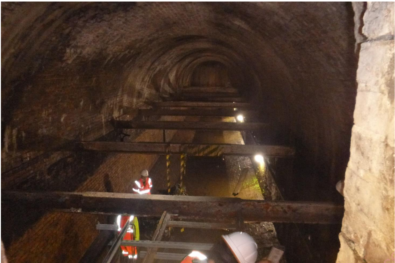
Figure 8 – The vaults of the coal stores with the wrought-iron beams across the vault
