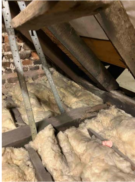
Fig. 6 : Strapped & re-supported loft beam
