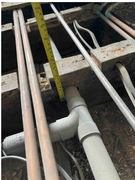
Fig. 3 : Notching to existing floor joists
