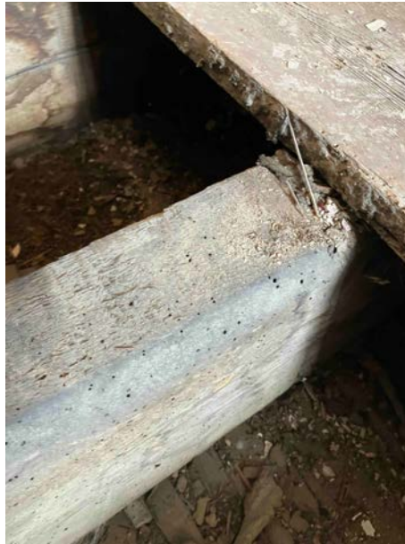
Fig. 2 : Woodworm to existing joists
