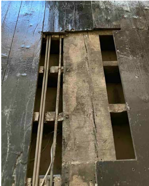
Fig. 1 : View of main floor beam / joists
