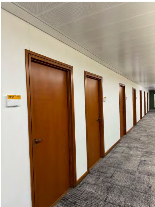
Typical corridor view across 2 nd , 3 rd & 4 th floor corridors - post refurbishment (2022/5402/L) New FD30 flush panel doors, stained finished to match refurbished retained door frames, architrave & skirting
