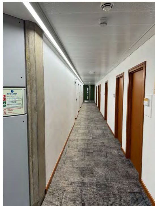
Typical corridor view across 2 nd , 3 rd & 4 th floor corridors - post refurbishment (2022/5402/L) New FD30 flush panel doors, stained finished to match refurbished retained door frames, architrave & skirting
