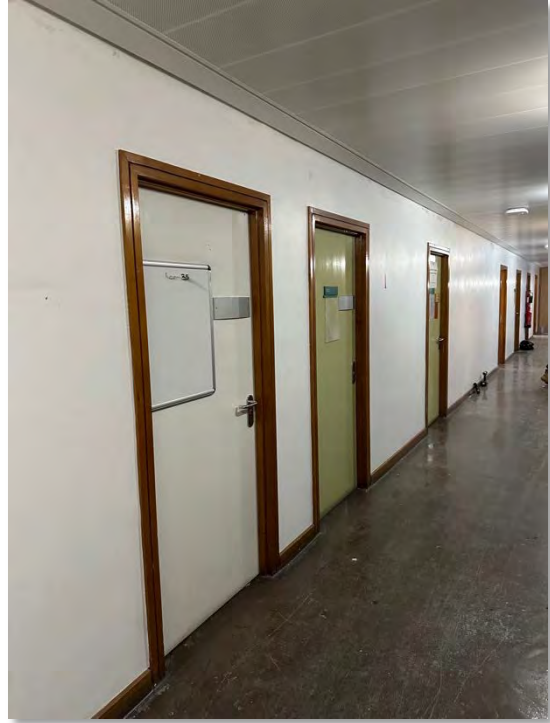
3 rd Floor Typical corridor view pre refurbishment Office/teaching room decorated flush panel doors with stained hardwood frames, architraves & skirtings
