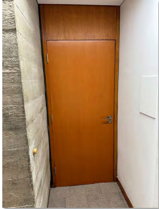
New FD30 flush panel door with fixed panel over, stained finished to match refurbished retained door frames, architrave & skirting
