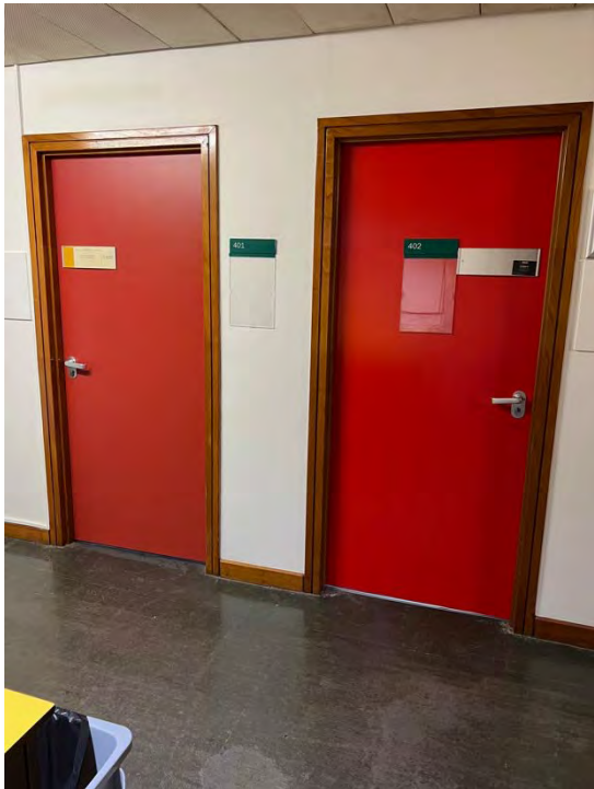
4 th Floor – pre refurbishment Office/teaching room decorated flush panel doors with stained hardwood frames, architraves & skirtings
