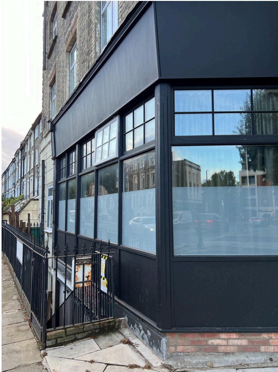
Front view of the site (93 Agar Grove)
