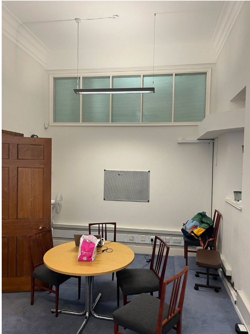
Fig. 28: Partition wall with wired glass, from office G01
