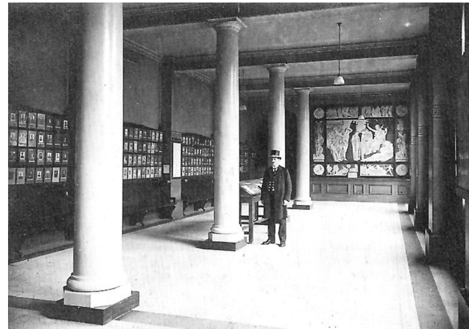
Fig. 18: The South Cloister in the inter-war period. Wilkins original columns would not survive the Second World War and the consequent rebuilding.
