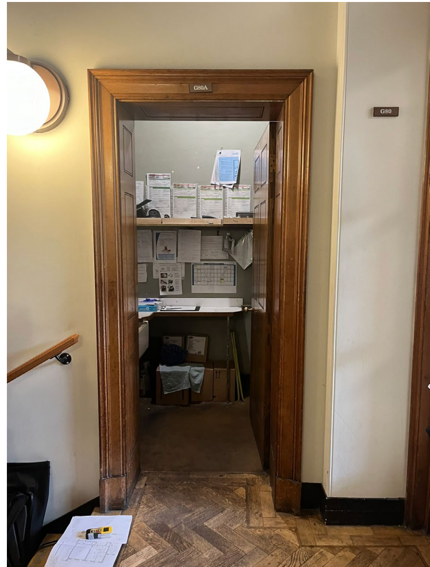
Fig. 32: Door architrave to store cupboard (Room G80A)
