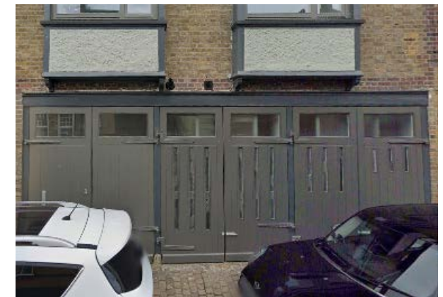
Figure 10. Example of similar cut-outs in Garage doors at no. 12 Daleham Mews, NW3.
