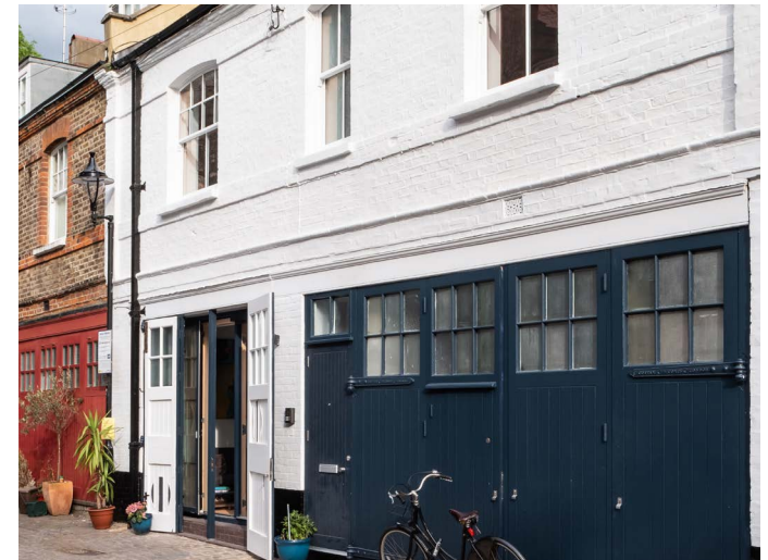
Figure 3. Front elevation of no.4 with characteristic features retained.
