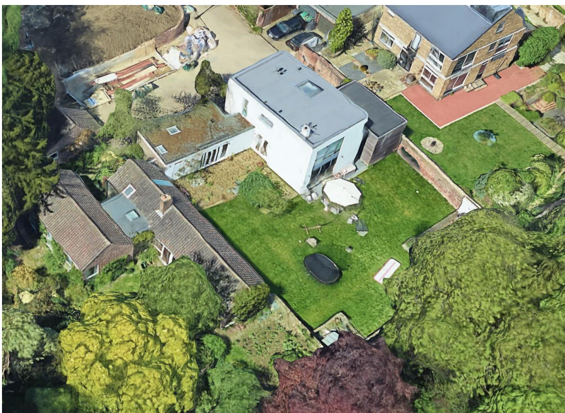
Figure 4.1 The application site
