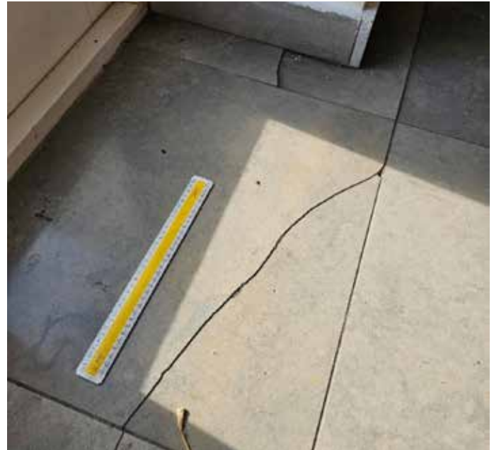
Photograph of cracks in floor showing ongoing building movement.
