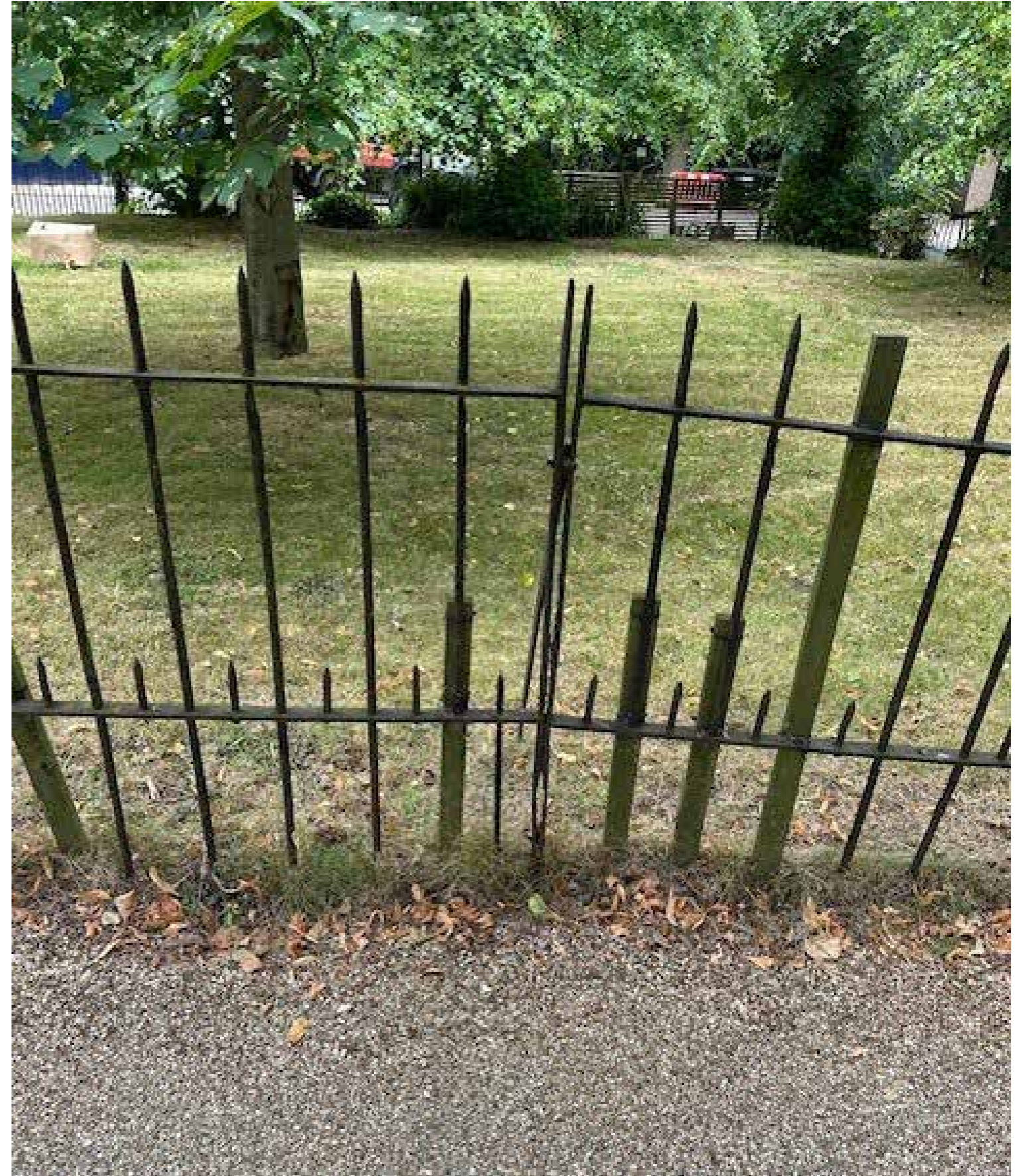
6. Panel with missing upright and dog rails
