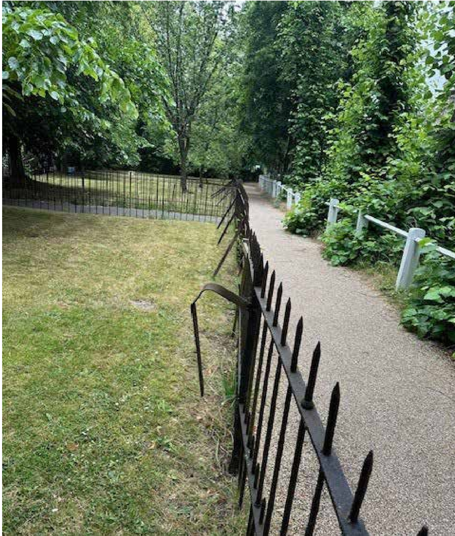
13. Damaged strut
