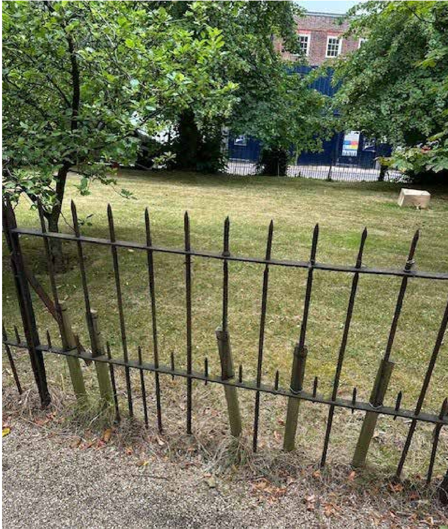
7. Panel with missing dog rails replaced
