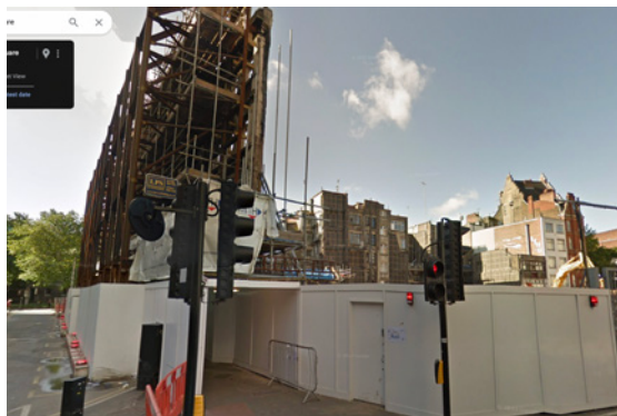
2016 street view - facade retention
