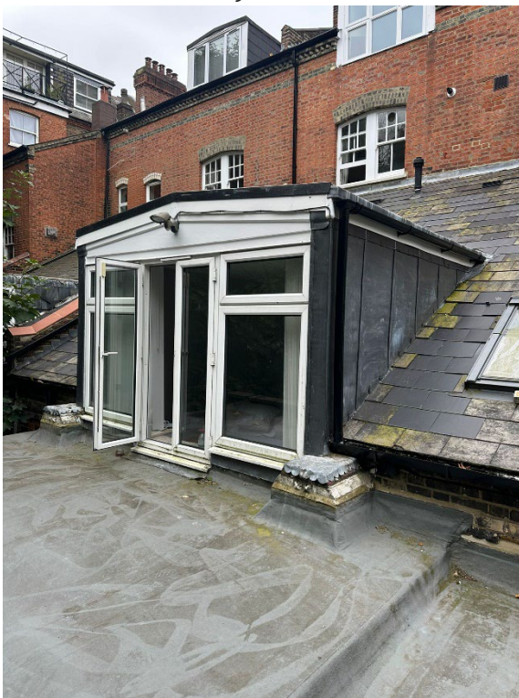
Photo above left: First floor roof terrace via Bedroom.
