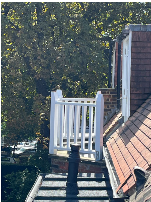
Rear bay railings at 2 Windmill Hill
