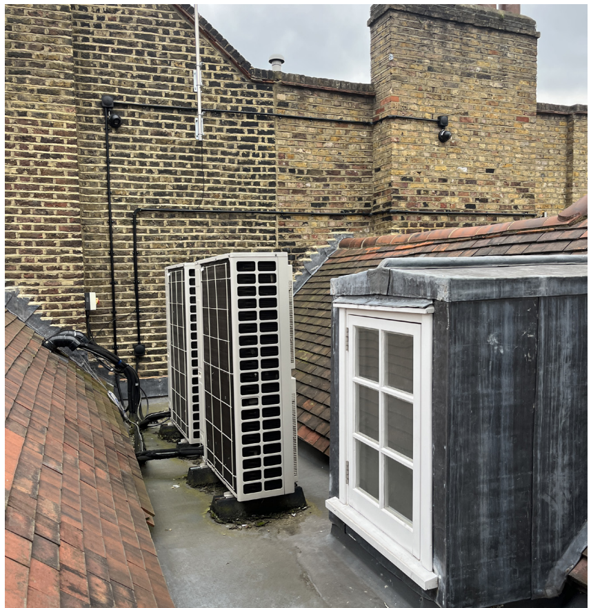
Air conditioning units to roof of No.40 Great James Street
