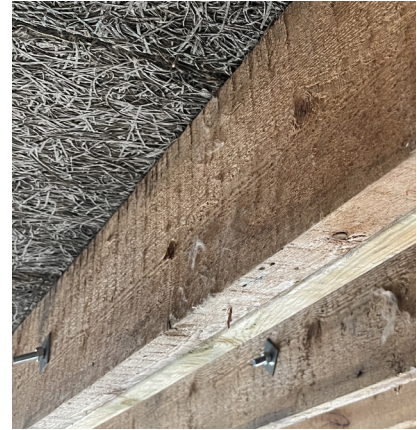
Modern third floor ceiling joists with visible saw marks
