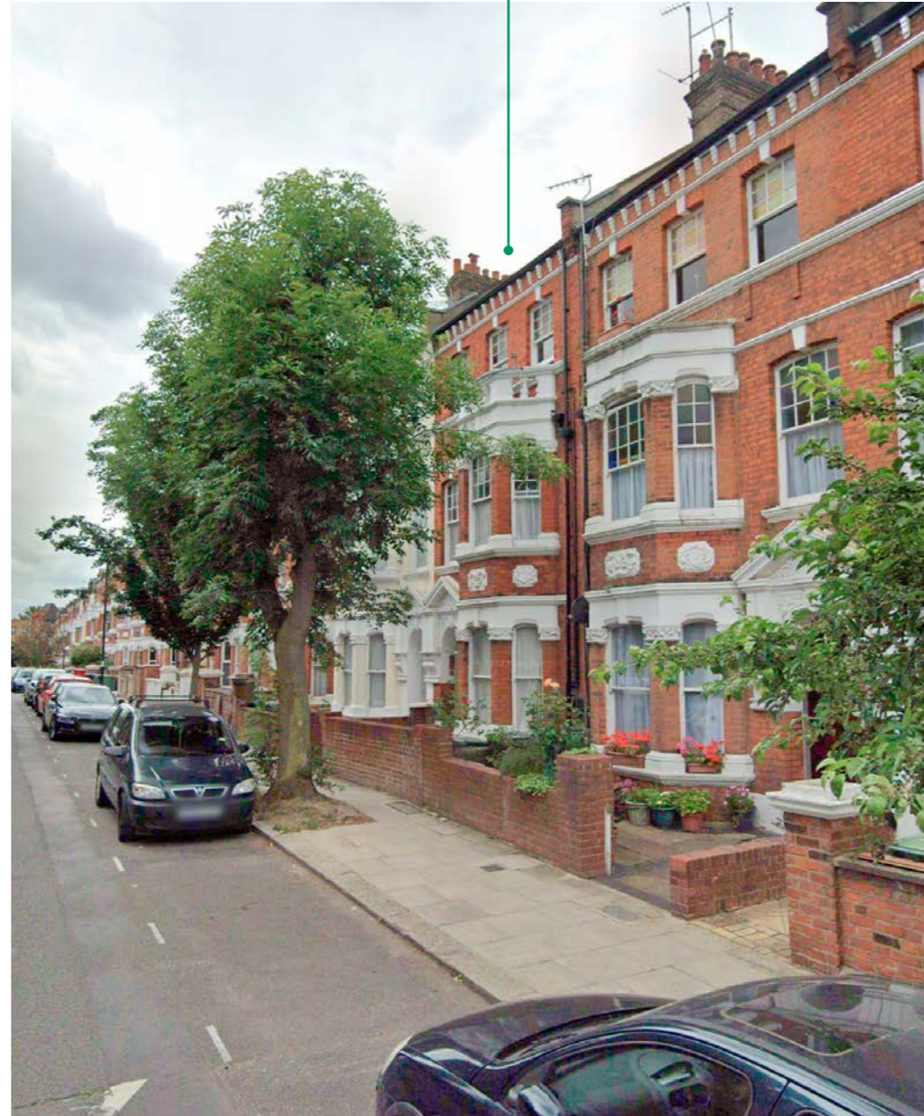
Street View of 48 Mazenod Avenue
