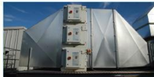
3 ESP Units Stacked in modular formation
