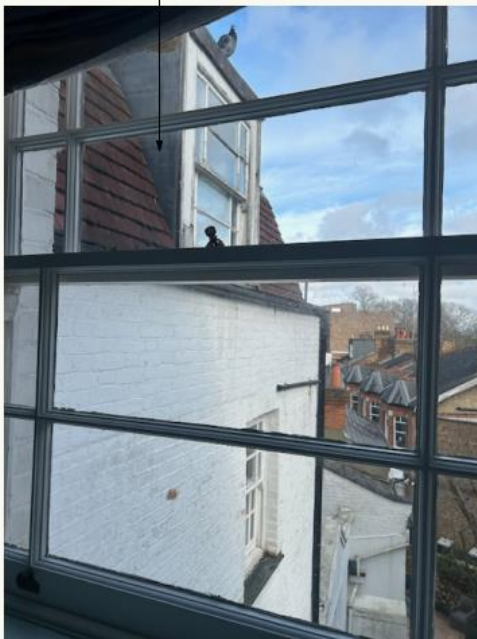
Non-original dormer window extension (existing)
