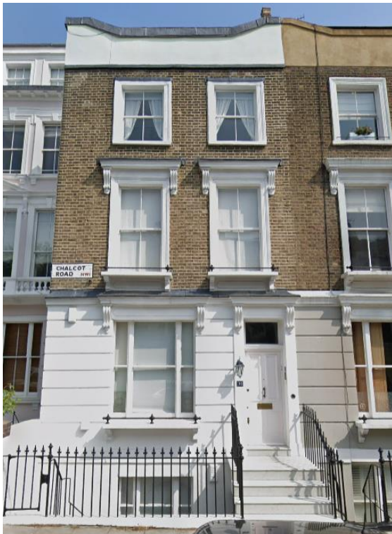
Images 1 & 2: Photographs of front and rear elevations
