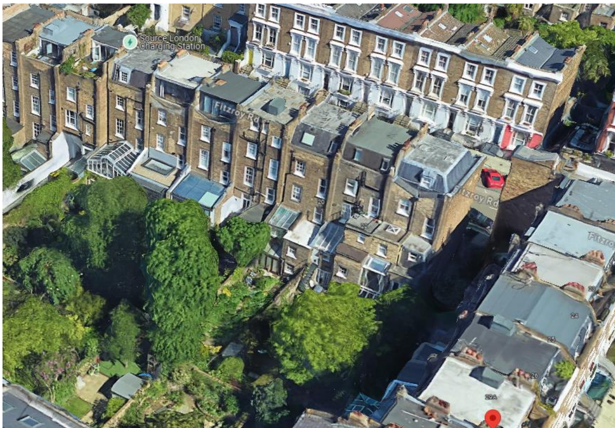
Image 4: Aerial view towards Fitzroy Road to East
